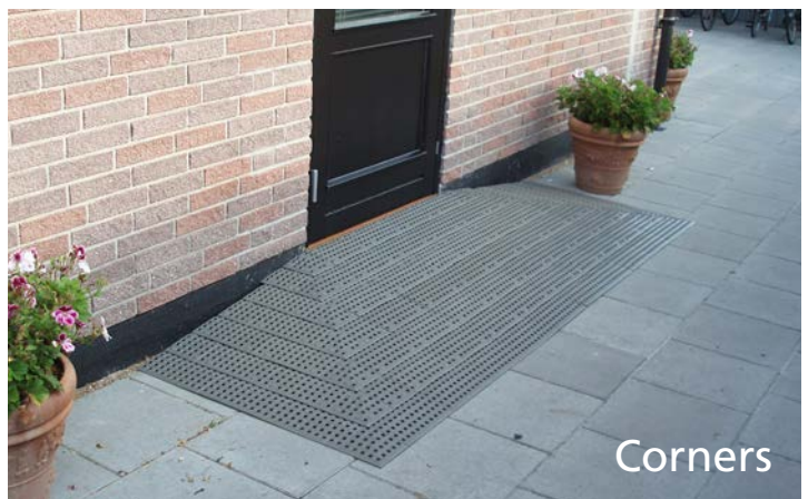
Corner ramps provide access from every angle. They have no edges to trip over and can be driven on by vehicles.
