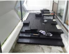
This balcony is raised approx. The floor is being raised and grey tiles are laid on top.
