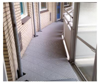
The floor of a narrow balcony access is being raised, thus creating optimal access to all flats. The floor is built up in several layers to facilitate its adaption to the building.
